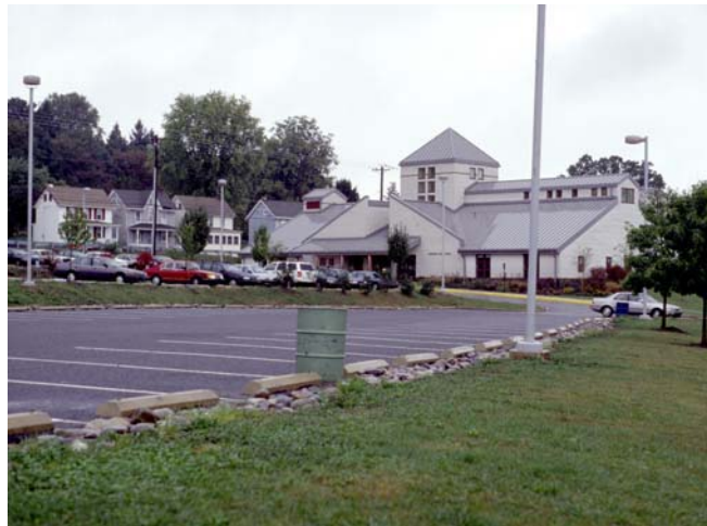
Figure 6.1-4 Porous asphalt parking lot at the Hockessin Library, Delaware (CA, 1991)
