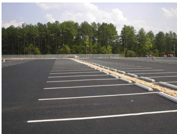
Figure 6.1-5 Porous asphalt parking lot at the University of North Carolina, Chapel Hill (CA, 2001)
